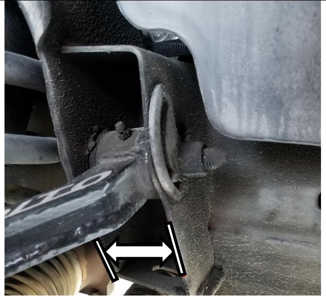
Figure 3: Factory Frame Service Perch Removal - After
